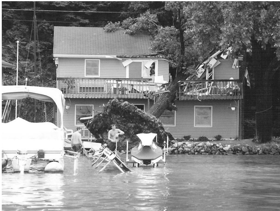
The Harman house after a 1997 storm dropped the tree ...
