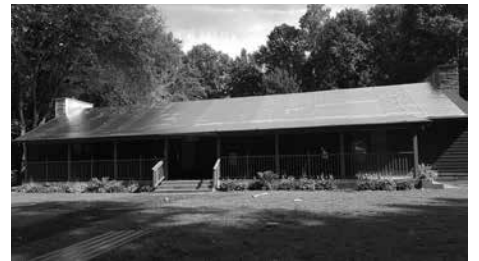
Dining Hall - In Progress
