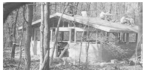
Candy Hill cabin under construction in 1975
