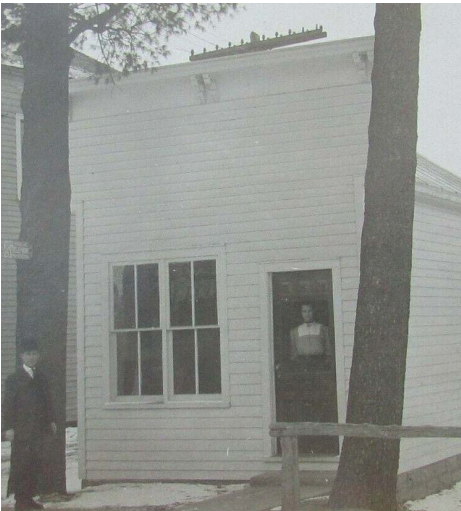
Perry Storey's Birch Lake Telephone Exchange, located in Williamsville
